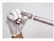
Assemble fitting on tube: To assemble the joint, the tube must be inserted into the fitting up to the tube stop. (Use the mark on the tube which was made earlier as reference). The pressing operation should only be undertaken when the tube reaches the tube stop.
