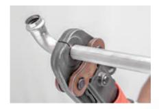
Press joint: Initiate the pressing procedure by pressing the start button for approximately 3 seconds. The pressing procedure will run automatically and should not be interrupted prematurely. This ensures a permanent joint that is sealed and has the required tensional and axial force locking properties. After completing the pressing process, the pressing tool can be removed from the pressed connection by opening the press jaw.
