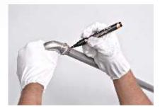
Marking the insertion depth: The tube must be fully inserted into the fitting until it reaches the tube stop in order to make a perfect joint. Marking insertion depth will ensure that any tube movement is detected, which is especially important if the joints are to be pressed at a later time.
